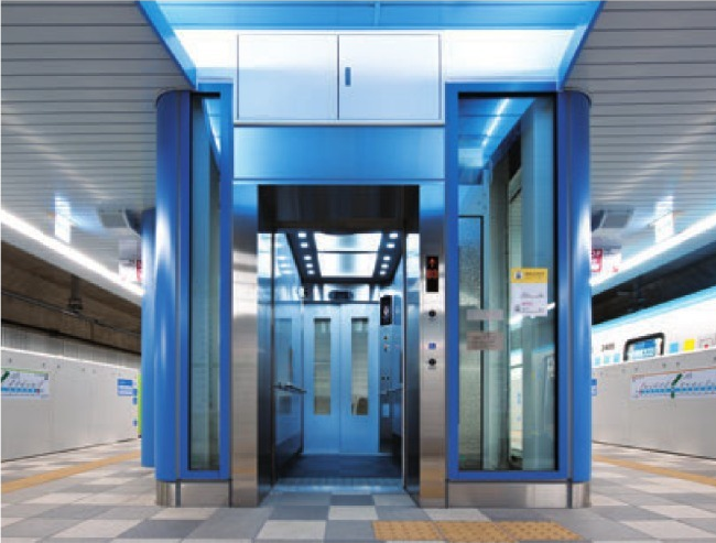
13-person passenger elevator (Yagiyama Zoological Park Station, train platform floor)
