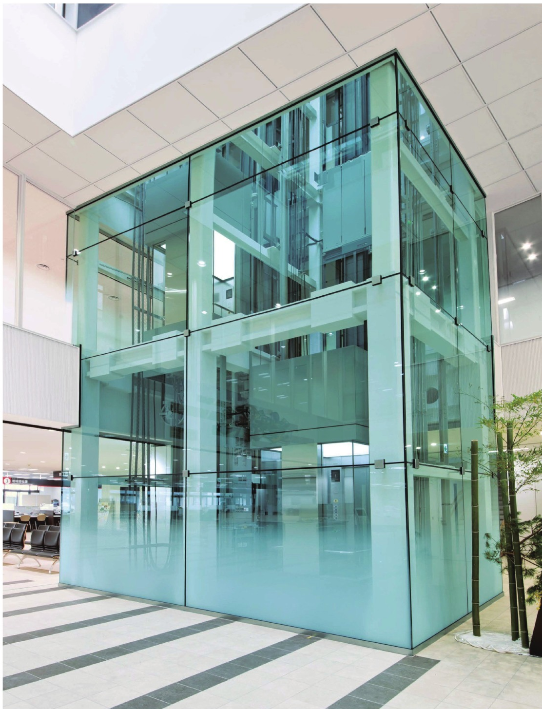
Observation elevator shaft
